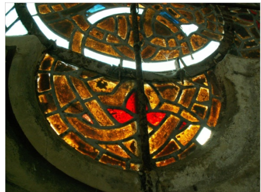
Fig. 4 Stained glass windows affected by browning, Abbaye Royale de Fontaine-Chaalis, France
